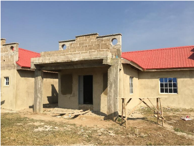
Plastering has begun on the Administration building
